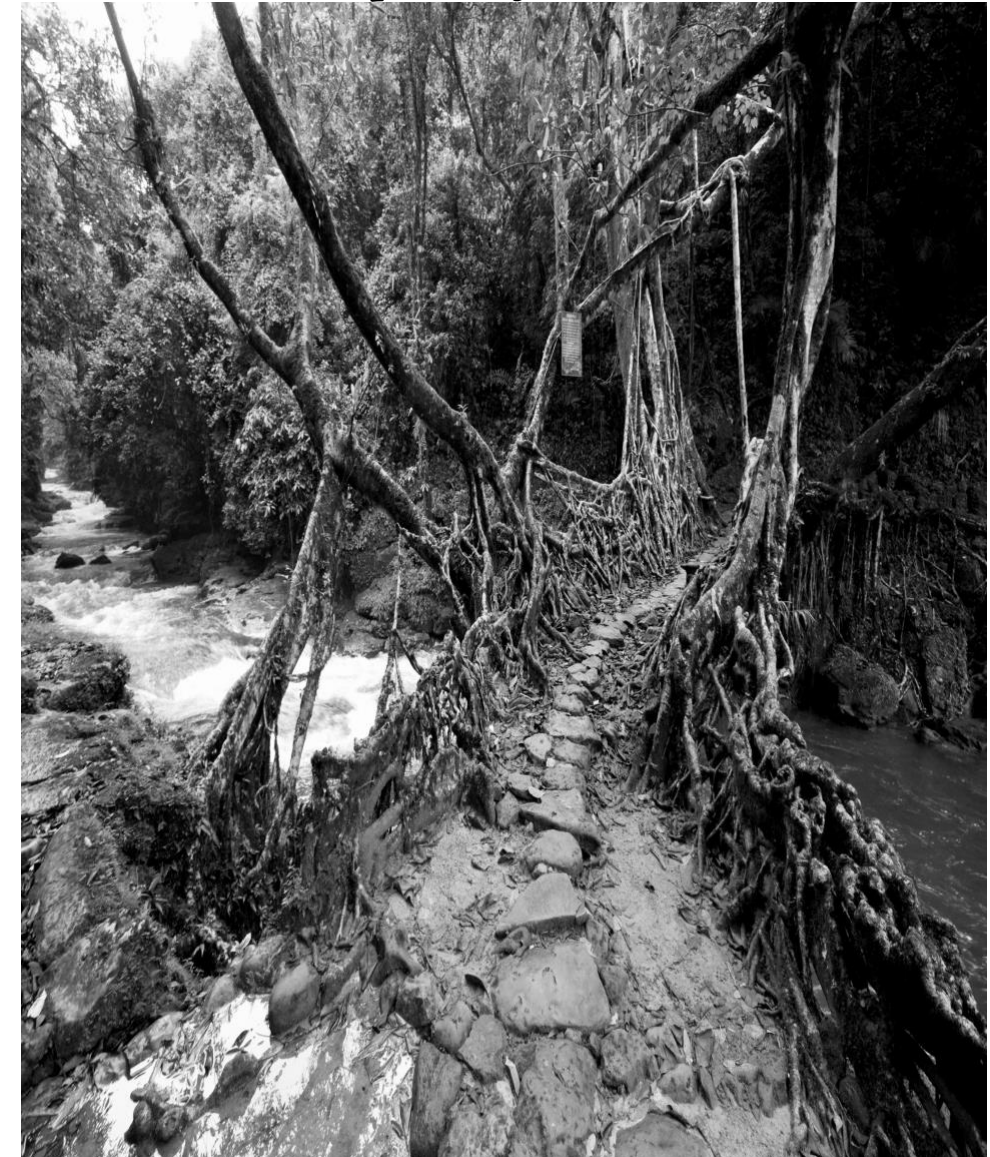
Meghalaya's Living Root Bridge
